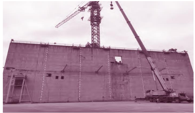
Figure 3: Rock impact test platform of a concrete retaining wall
