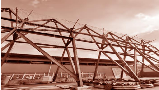
Figure 6 A steel structure rock fall impact test platform
