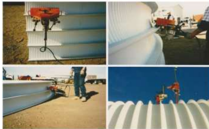
Figure 3 (K-Span Jointing) (A. Piekarczuk, 2021)
