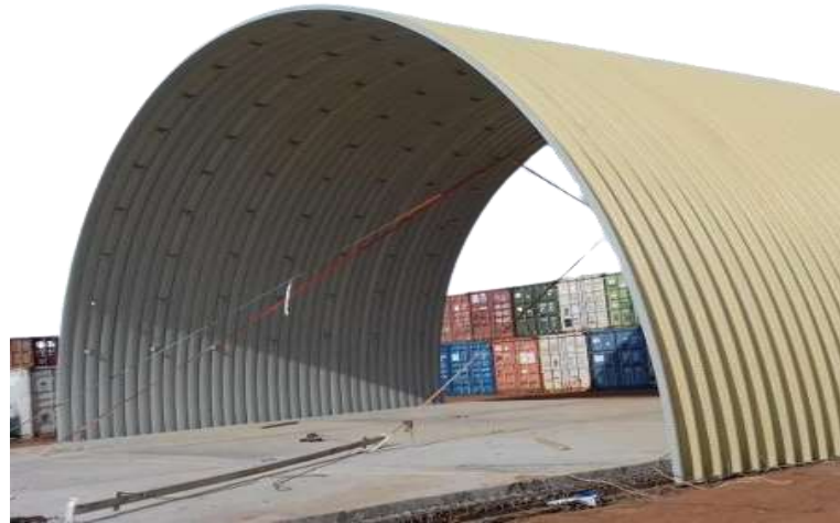
Figure 1: K-Span Structure (Artur Piekarczuka, 2019)
