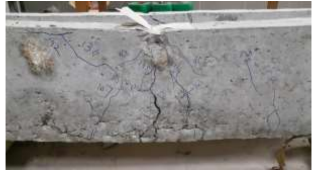
Flexural Cracking of Beam at 60° Angle
