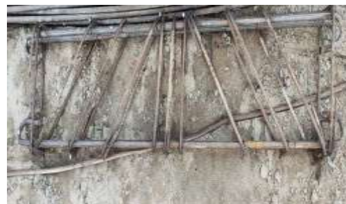
Steel reinforcement at 45° Angle
