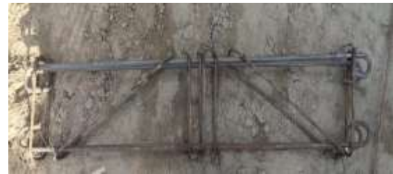
Steel reinforcement at 30° Angle
