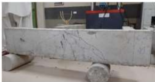
Cracking of Beam at 90° Angle
