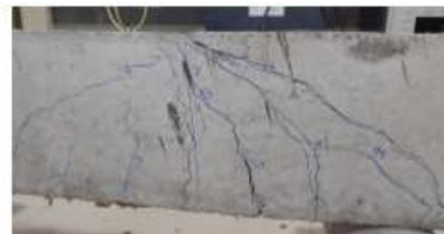
Flexural Cracks of Beam at 90° Angle
