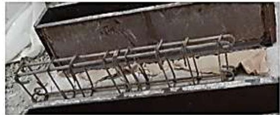
Steel reinforcement at the 90° Angle
