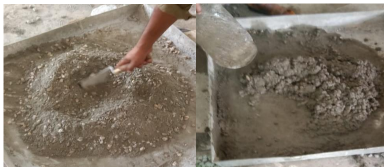
Figure 2 Mixing of concrete
