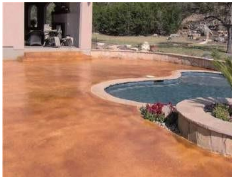
An acid-stained Pool deck floor
