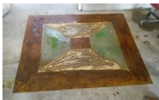
Applying iron sulfate, copper sulfate, copper chloride, and sodium sulfate acid stain solutions to the laboratory floor at Building & Architectural Engineering Department BZU Multan.
