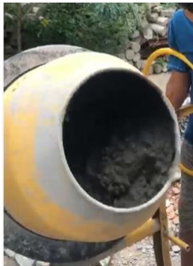
Fig. 1 Mixing of concrete ingredients in a tilted drum mixer
